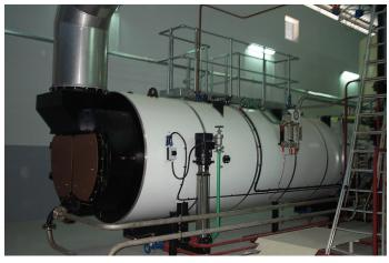
The waste heat from the oxidisation chamber passed through a waste heat recovery unit – incorporating a super heater bank and shell and tube design boiler (the project supply included the water conditioning plant).
