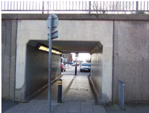
The pedestrian underpass is the most direct link from the bus stop on south way to the High Street/Newhaven Square.
