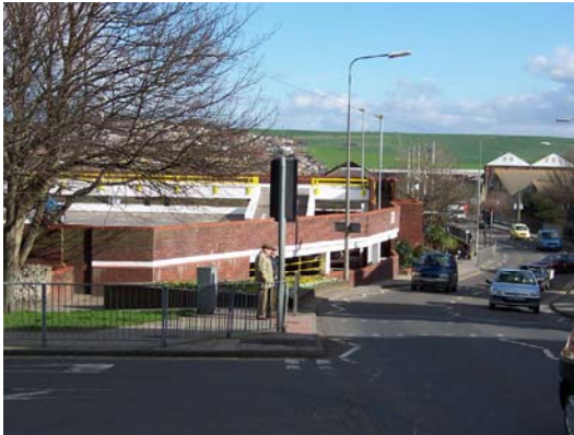
Multi-storey car park along the southern edge of the town centre presents a poor image to those passing on the ring road
