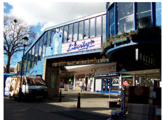
Insensitively designed modern additions with large signage and garish colour schemes
