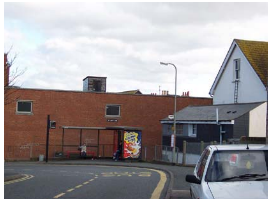
The bus stop in North Lane offers a bleak view of the town centre.
